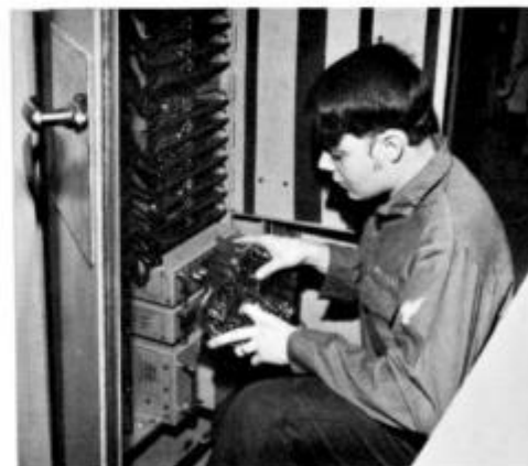
IC3 Hoffman expertly replaces an electrical board.
